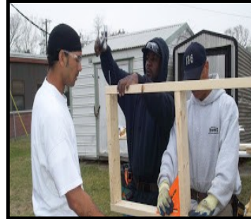
Basic Construction Skills
