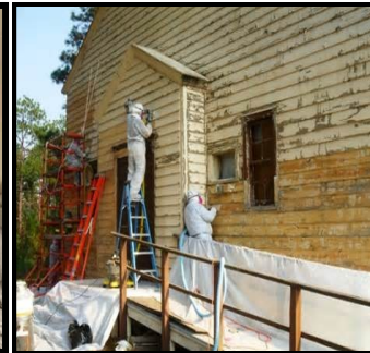
Lead Paint Abatement
